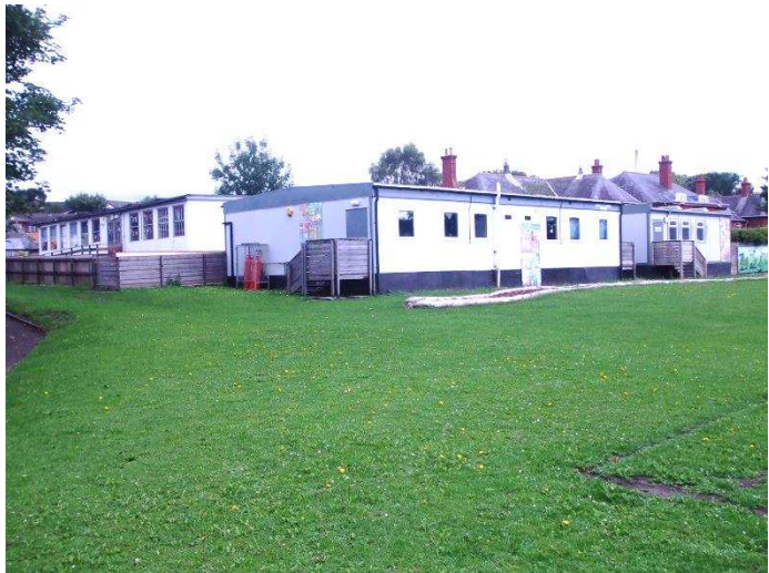
Ysgol Pen Barras mobile classrooms
